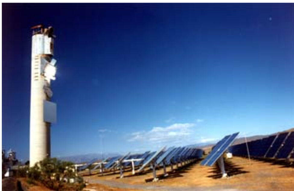
Figure 4: Experimental central receiver system at the European research center Plataforma Solar de Almería in Spain
