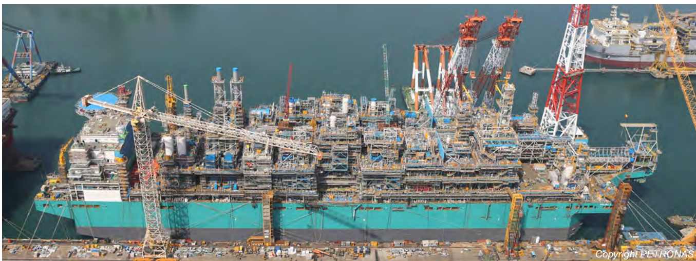
The PETRONAS FLNG SATU has been completed and is expected to commence production in 2016. Photo courtesy PETRONAS.
