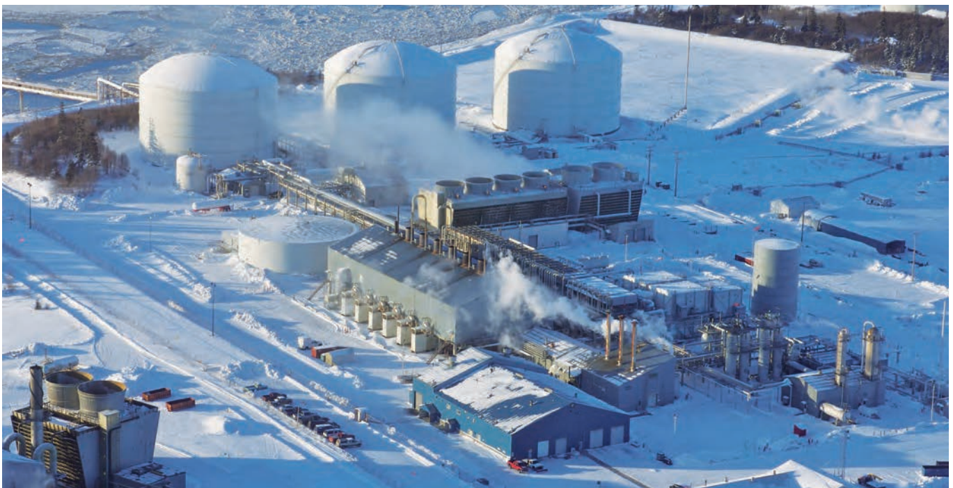
Kenai plant. Photo courtesy ConocoPhillips.
