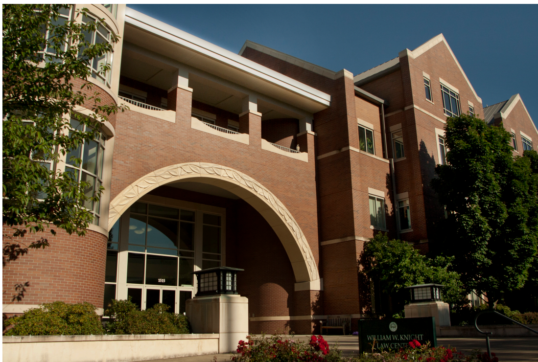
Knight Law Center is one of two buildings trying for LEED Certification of Existing Buildings. It won't be approved for certification until August of 2012, but preliminary data collection has begun.
