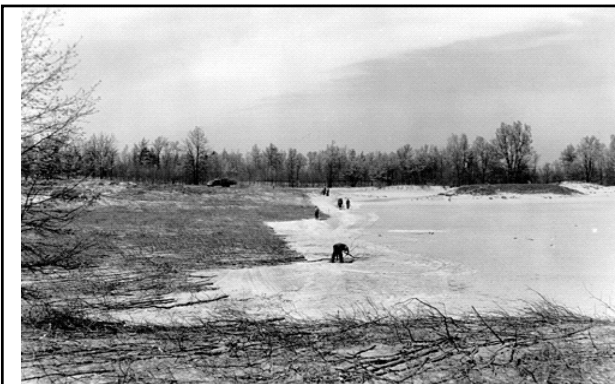
Resettlement Administration Submarginal Land Purchase in SW Michigan. Relief workers combat soil erosion by covering failed farmland with branches.
